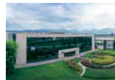
The New Factory
