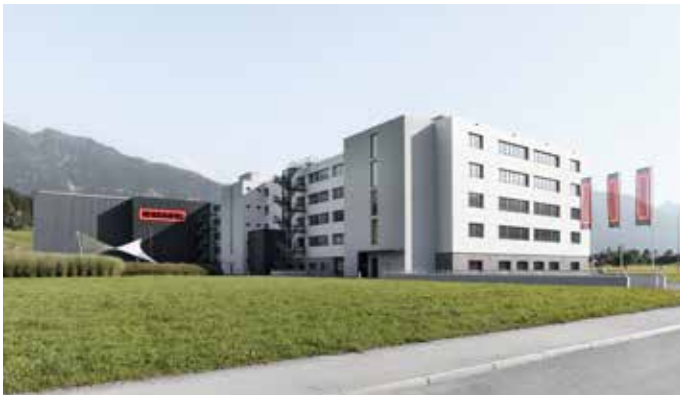
Leister Technologies AG, factory, Samen, Switzerland
