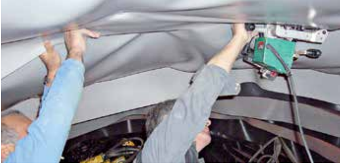
Comet operating in the tunnel ...
