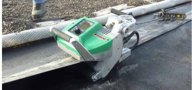
The GEOSTAR easily welds 240 m without difficulty in a single pass during a field test (South Africa)..
