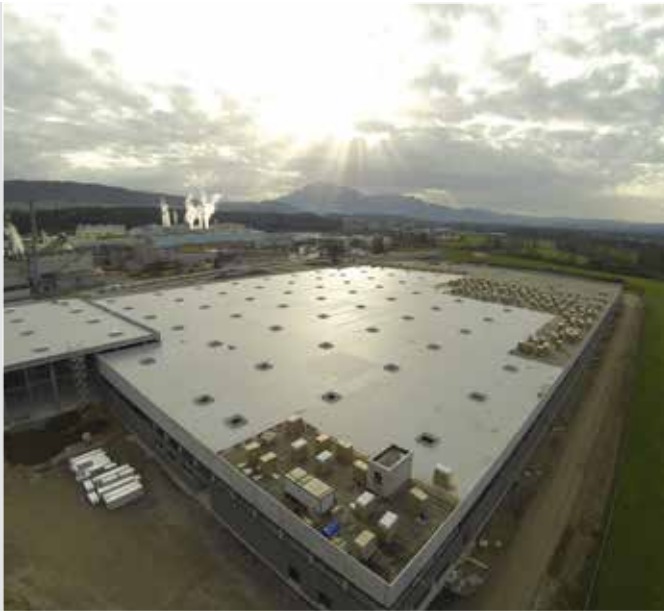
Aldi logistics center 50000m2 TPO Membrane, Switzerland
