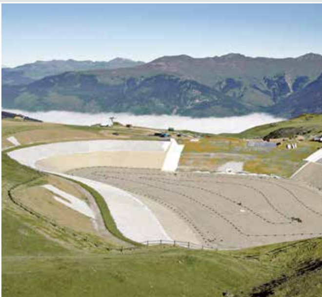
Water Reservoir HDPE 2.0 mm
