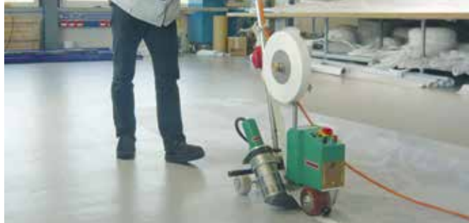
Welding tape at maximum speed.
