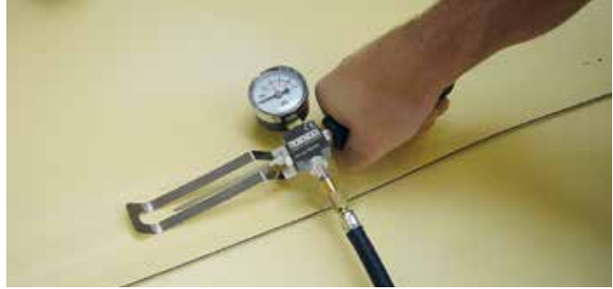
Testing the leak-tightness of lap seams with test channel.
