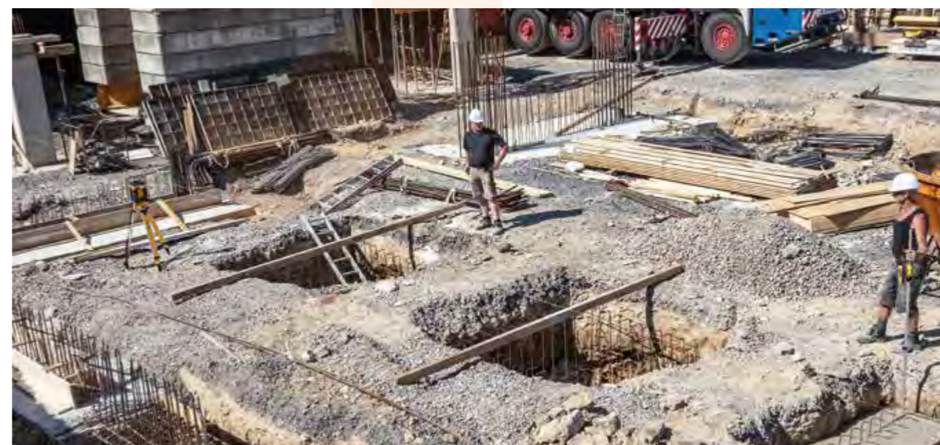
The laser is impressively easy to operate and, when used together with the REC 300 Digital receiver, allows tasks to be carried out rapidly and reliably within a working area of up to 800 m.
