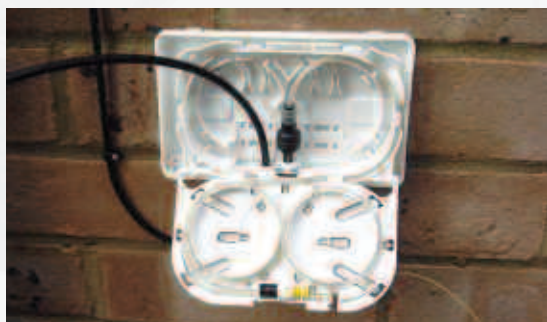
Typical use of a John Guest Gas Block/Fibre Lock & Straight Reducing Connector in a customer splicing point enclosure.
