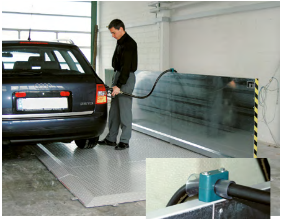
Compact fuel dispensing area
