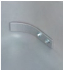
Platform fastening (reinforcement)
